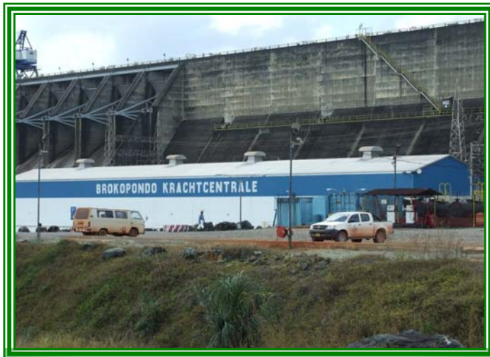
Hydro-power facility at Brokopondo
