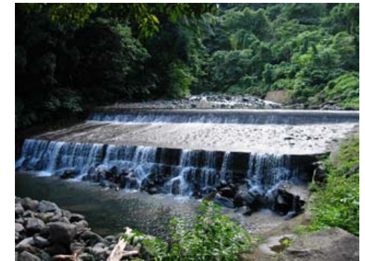
Dam for Hydropower Plant at Richmond, St. Vincent
